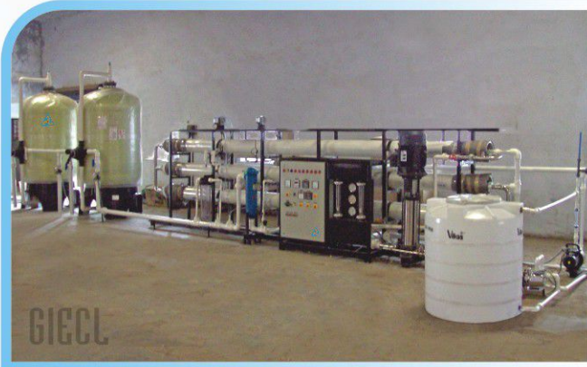
25.0 M3/Hr R.O. System for Brackish water for Drinking installed in Mauritius
