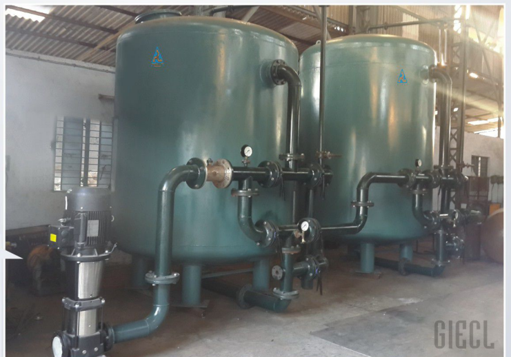
2.0 M3/Hr HSRO System with EDI system for Ultra High Purity Water for Pharmaceutical industries for USP, EP, WFI standard
