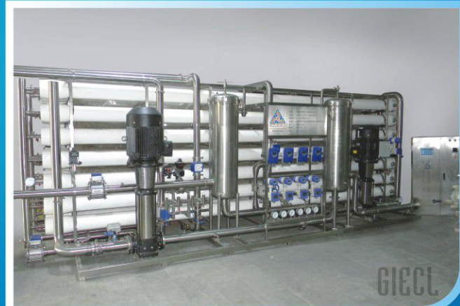
67.0 M3 /Hr First Pass and 50.0 M3 /Hr Second Pass Fully Automatic Most Advanced featured RO System for ultra pure water generation using ultra sonic flow meters, online pH & TDS controller, VFD driven Grundfos Pump with full HMI Controlled PLC Panel
