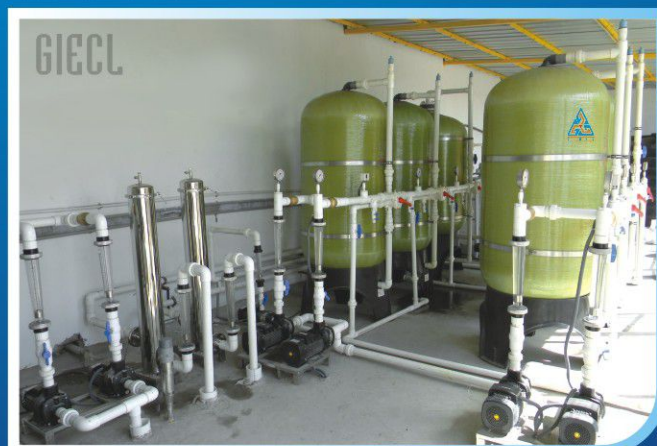
15.0 M3/ Hr. Water Filtration Plant for Township and communities supply
