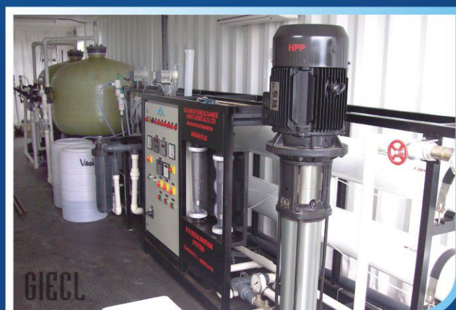
10.0 M3 / hour Sea Water De Salination plant used for civic supply on island for drinking and house hold application with mobility use
