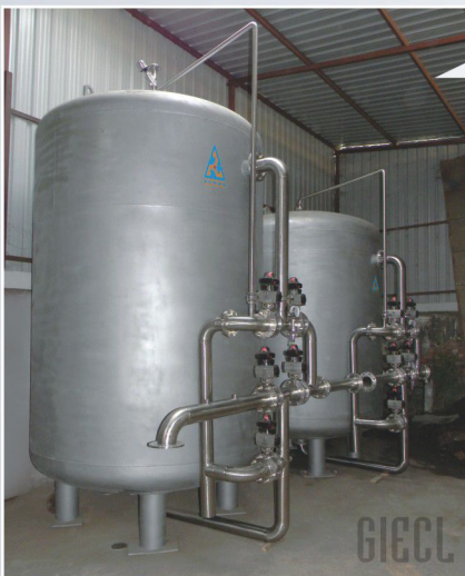
3.0 M3/Hr Two Pass R.O. System with Ultra Pure water production for Pharmaceutical factory
